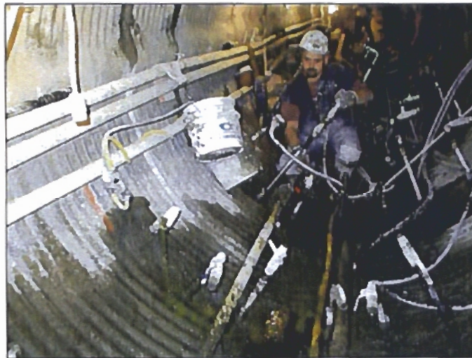
Figure 6. Permeation/fracture grouting and compensation grouting at CMP.
