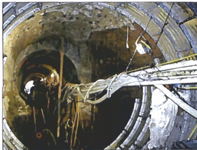
Figure 8. Exposed soil surface after excavation at CMP.
